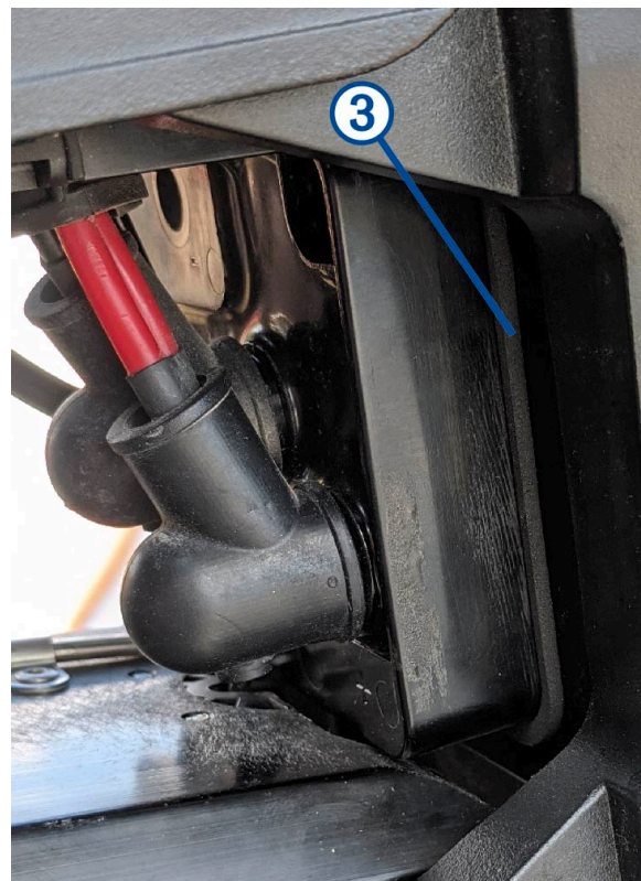
Motor with the Seal Installed
